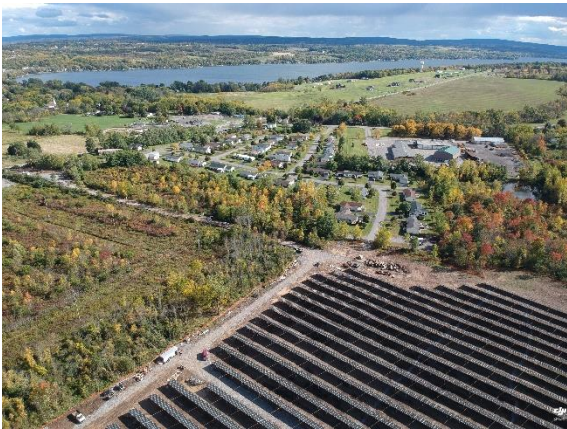
Lakeville Community Solar
