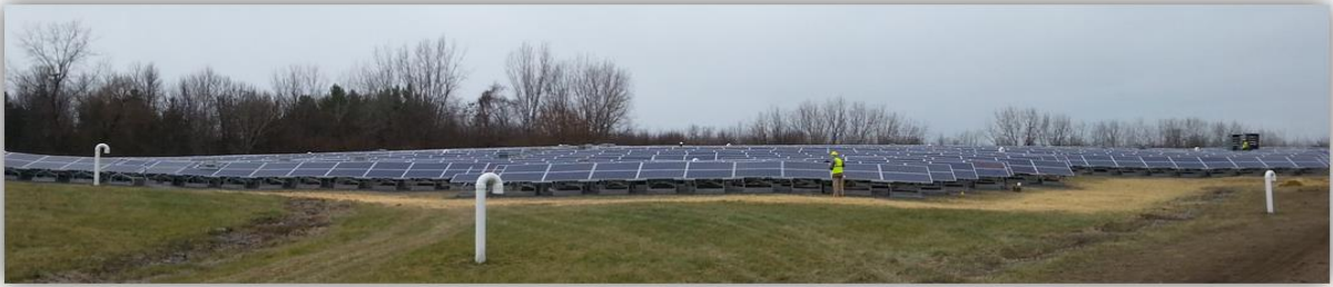
Town of Williamson – Wayne County, NY – Land Fill
